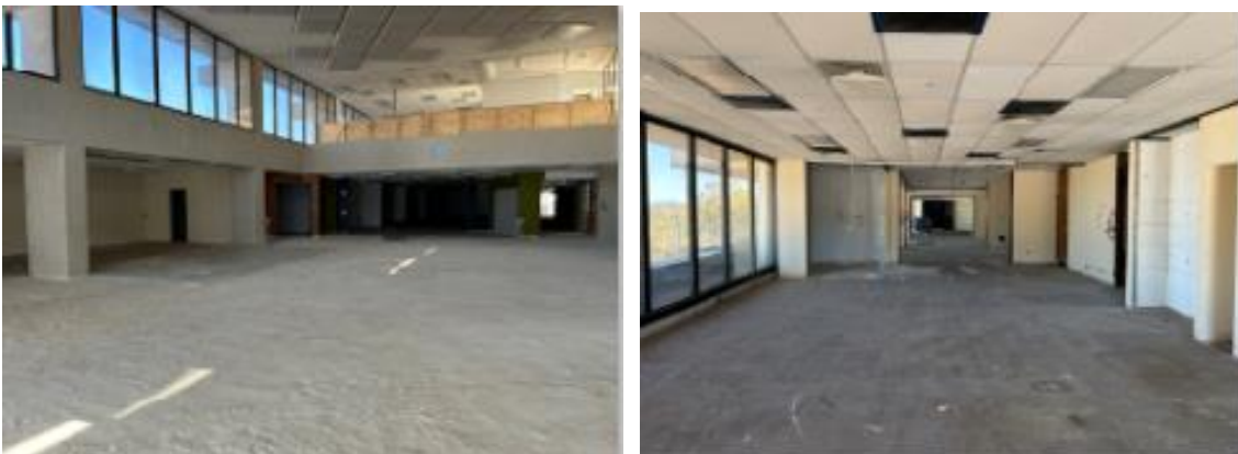
Images: Post Stage 1 Demolition
