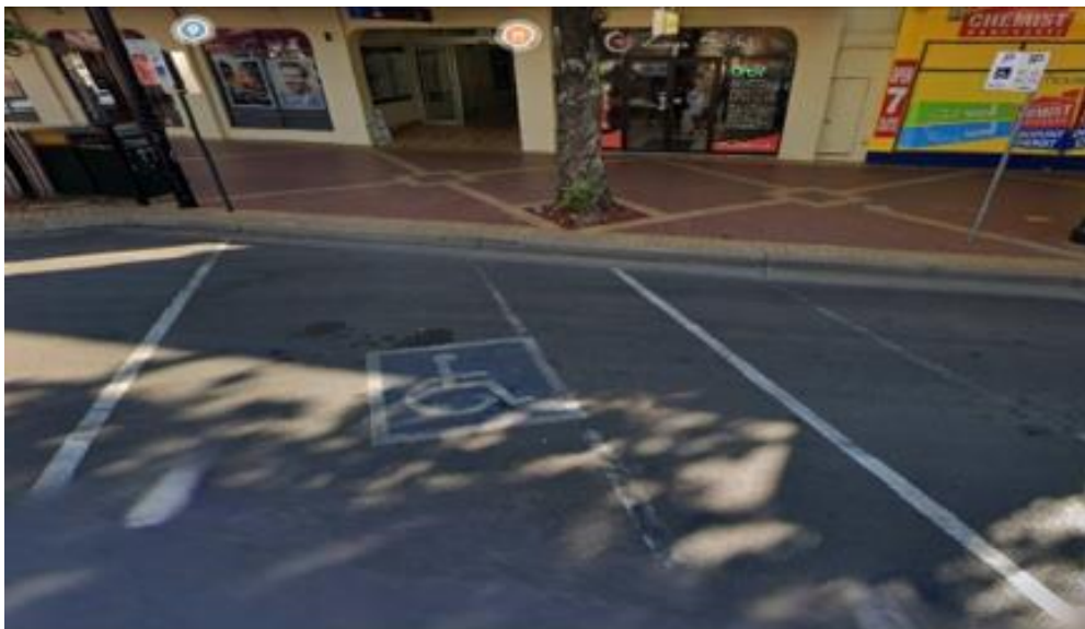
Figure 2: No kerb ramp associated with the two disability parking bays on Peel Street, Tamworth.
