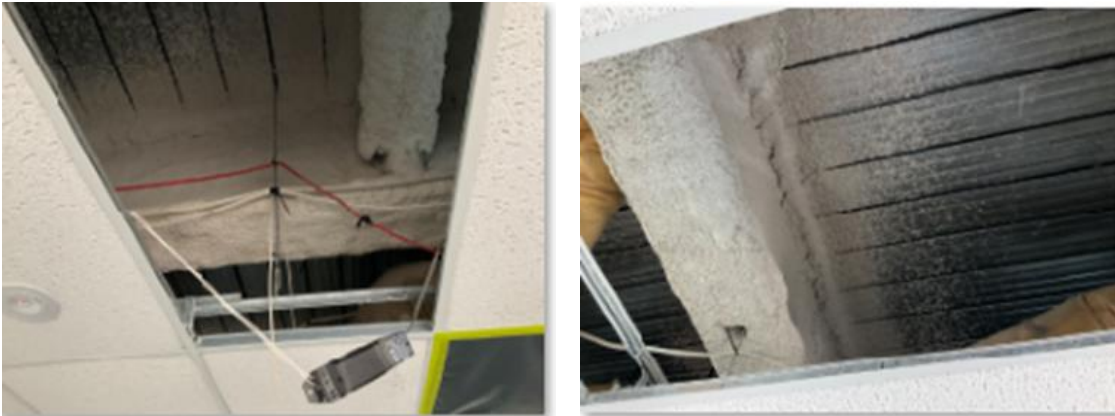
Images: Vermiculite in ceiling
